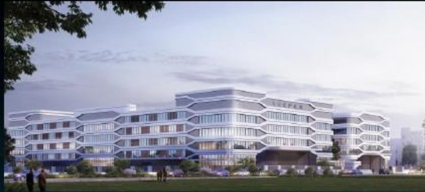
Phase 2 in construction
