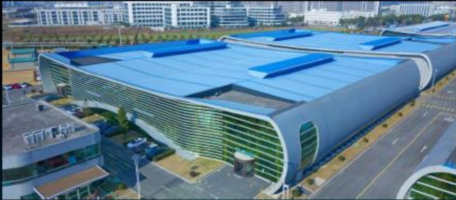
Phase 1 commissioned on Aug 15 th 2024
