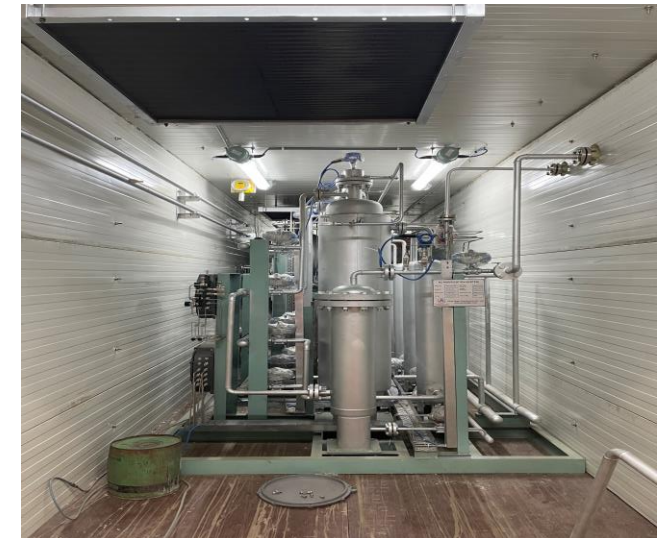
Electrolyser Container
